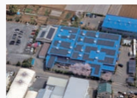
Factory rooftop, SHINANO INC.
