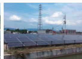
Wakayama Solar Power Plant
