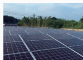
Kagoshima Solar Power Plant
