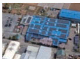
Factory rooftop, SHINANO INC.
